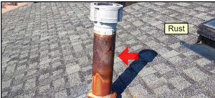
Chimney walls rusting or pitting
