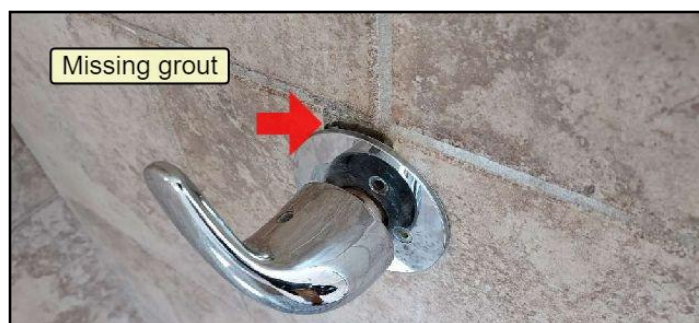
Grout loose, missing or deteriorated
