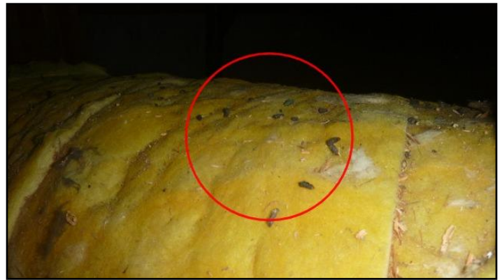
Animal/pest droppings in crawlspace
