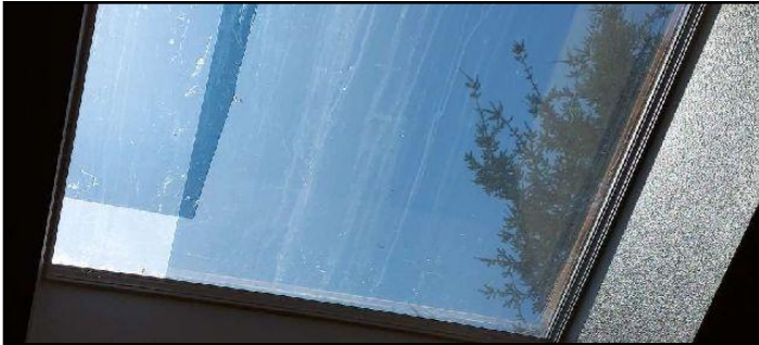
Lost seal on double or triple glazing
