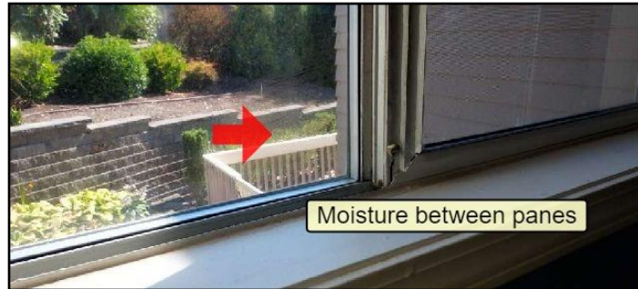
Lost seal on double or triple glazing
