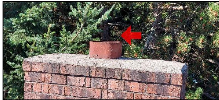
Spark Arrester Missing
