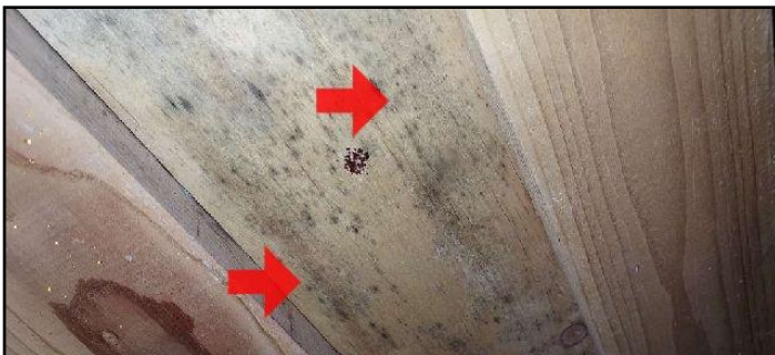
There is evidence of a mold-like substance...
