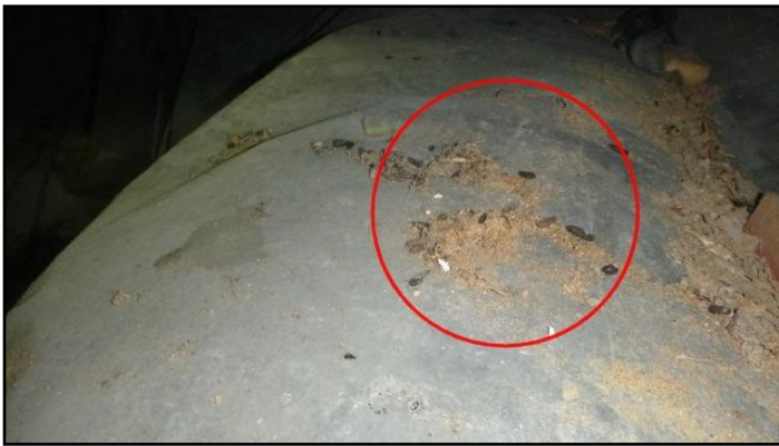
Animal/pest droppings in crawlspace
