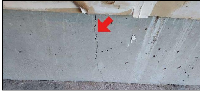
Typical minor cracks
