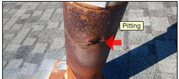
Chimney walls rusting or pitting
