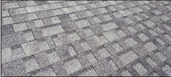
Asphalt shingles
