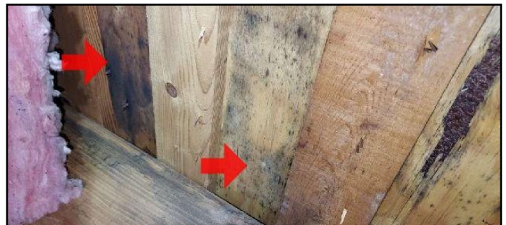
There is evidence of a mold-like substance...
